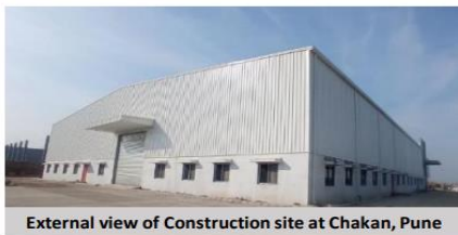
External view of Construction site at Chakan, Pune
